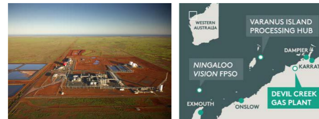
Figure 1 "Devil Creek Gas Plant Location Map and Aerial View"
